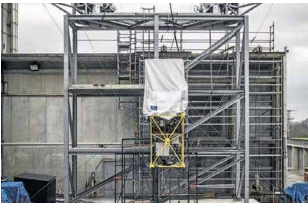
WE HAVE REDUCED THE RISKS ON WORK SITES USING CABLE ROBOTICS
